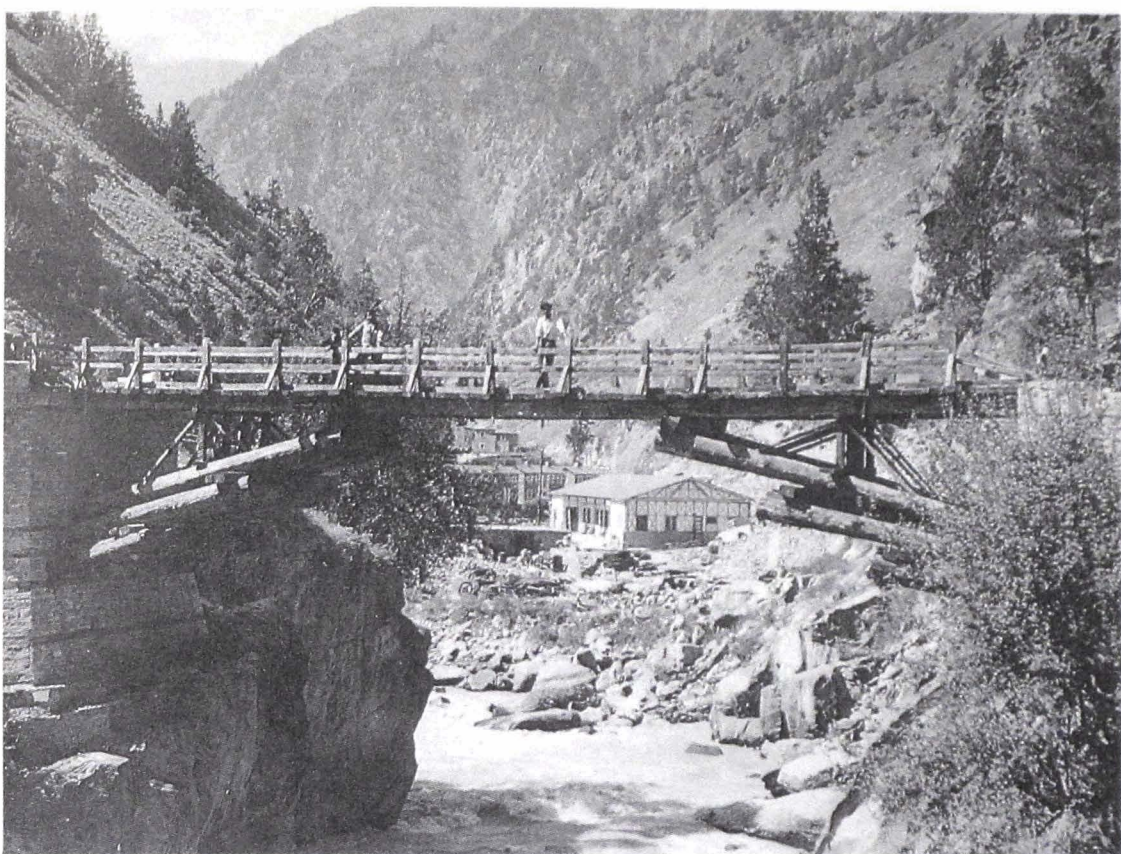
5. A cantilever wooden bridge, now a thing of the past.
